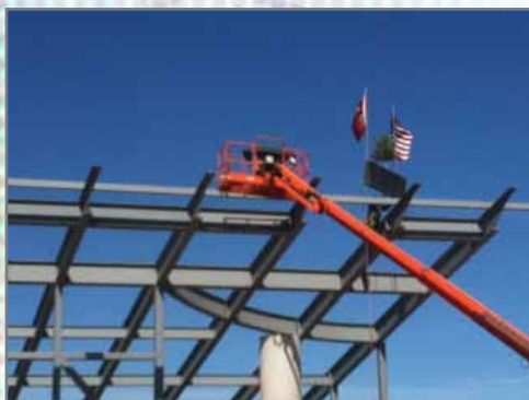
Beam being placed by crane
