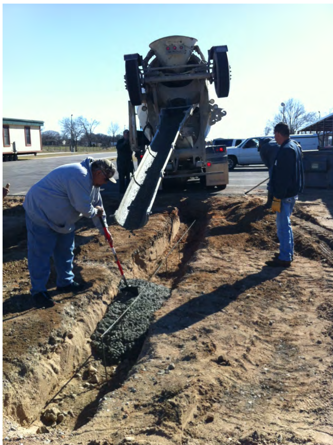
AST Maintenance Department pouring concrete
