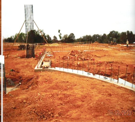
Main entry column rebar
