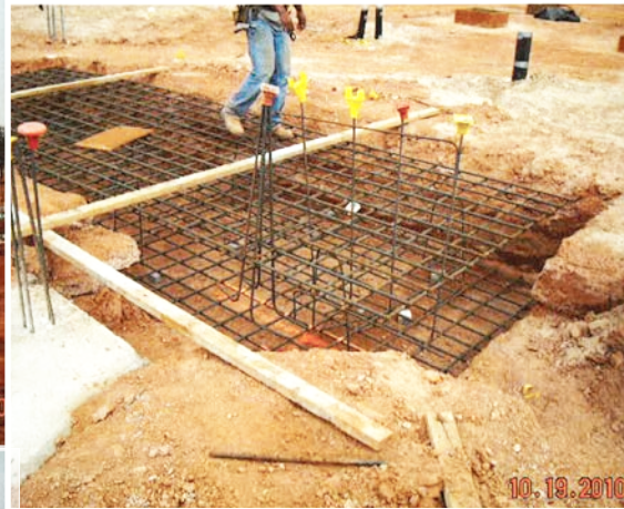
Working on spread footings
