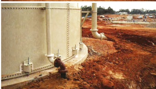
Tank supply piping
