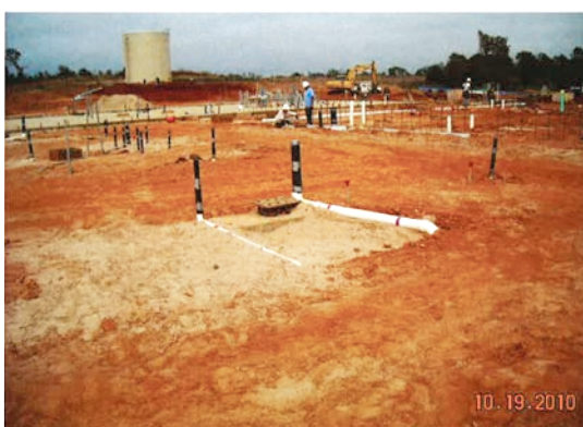
Working on prepping anchor bolts for steel erection
